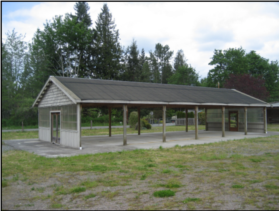
Existing Pole Barn As Picnic Shelter
